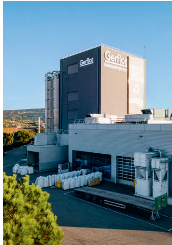
↑ Usine LVT, Saint-Paul-Trois-Châteaux, France.
